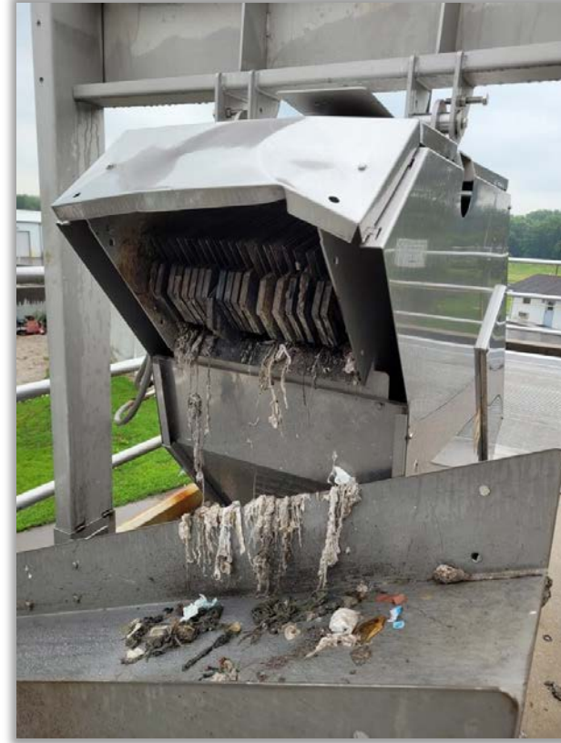
Wipes and Debris Clogging at WWTP
